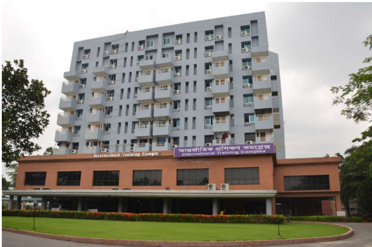
Front view of newly constructed ITC building of BPATC
